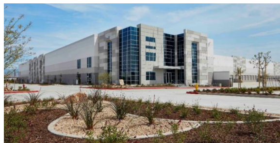
Ex: High level of building articulation, architectural elements, and textured materials reduce the visual impact of a long building façade.
