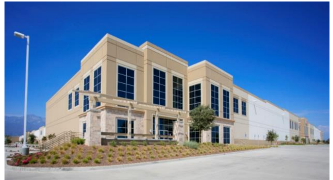
Ex: Secondary exposure side of a building architecturally compatible to the primary exposure of the building through use of windows and color blocking.
