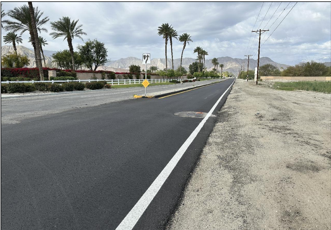
Figure 5-3 Overview of Avenue 50 opposite Verano Drive, facing west.
